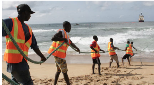
Fibre optic cable
